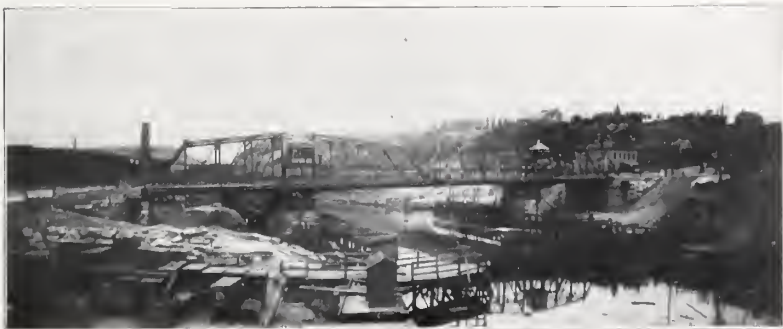
COLUMBUS STREET DOUBLE SWING BRIDGE The First of its Kind in the World
